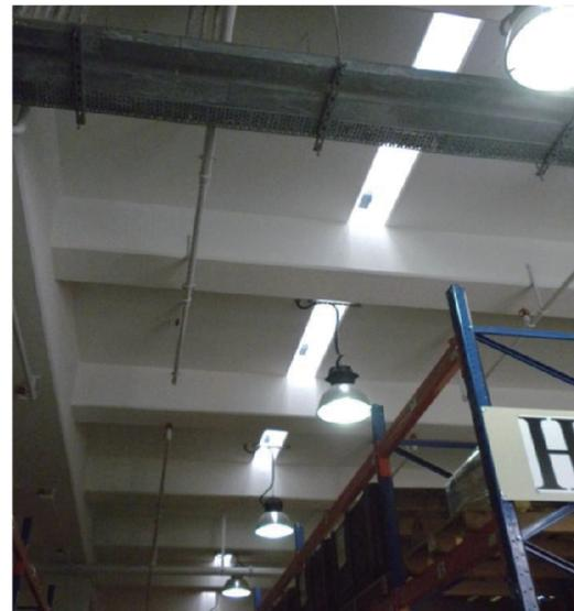
Fig. 2 thin strip of skylight added at regular intervals corresponding to the aisle location of each store
