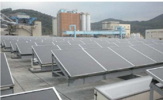
Fig. 2b TFPV Solar Panels on the roof of LMA East Store Building (side view)
