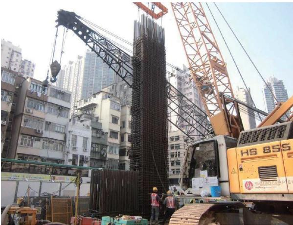
Figure 3 - Placing Steel Reinforcement Cage of Diaphragm Wall Panel
