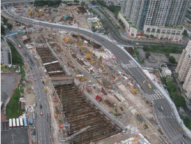
Figure 1 - Open Excavation at Urban Area
