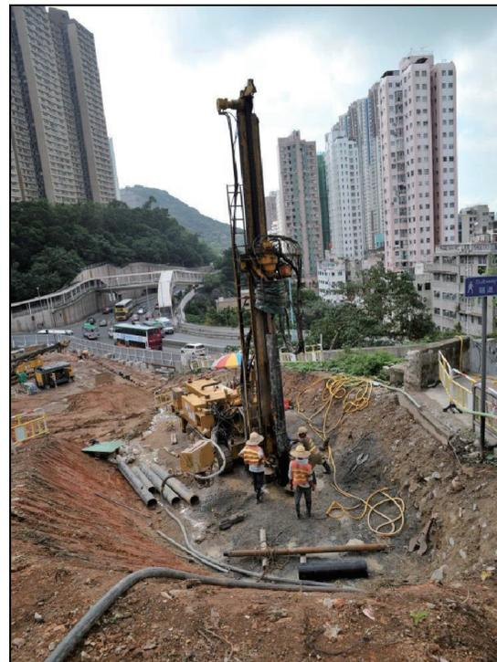
Figure 7 - Pipe Pile Installation by boring Method
